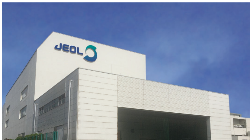
Akishima head office & factory
