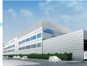
No.3 Akishima Head Office Plant (Enlargement of Clean Rooms)
