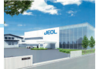
Tendo Plant in Yamagata Prefecture (YMCC)
